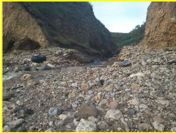
Erosion of beach crest by flow from beck at Ryhope Dene. (Locally active) (Asset ref. No. 121AB901B0804C02)
