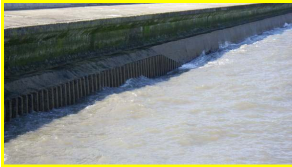
Toe piling to southern section crest wall. (Asset ref. No. 121AB901B0802C01)
