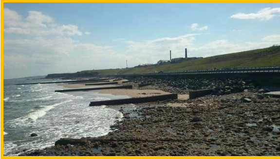
Concrete groynes on foreshore at Hendon (Asset ref. No. 121AB901B0803C02)
