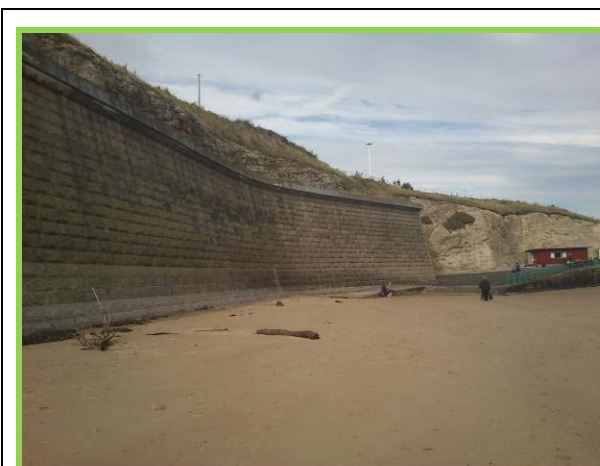
High masonry wall in good overall condition (Asset ref. No. 121AB901B0605C01)
