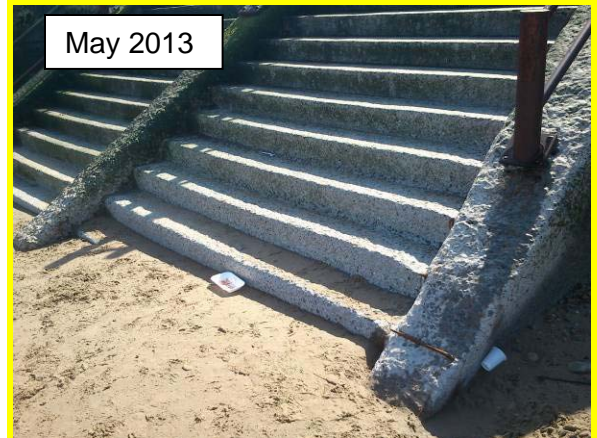
Abrasion of steps visible at low beach levels (Asset ref. No. 121AB901B0604C01)
