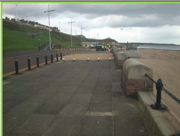
Resurfacing of section of promenade underway (Asset ref. No. 121AB901B0605C02)
