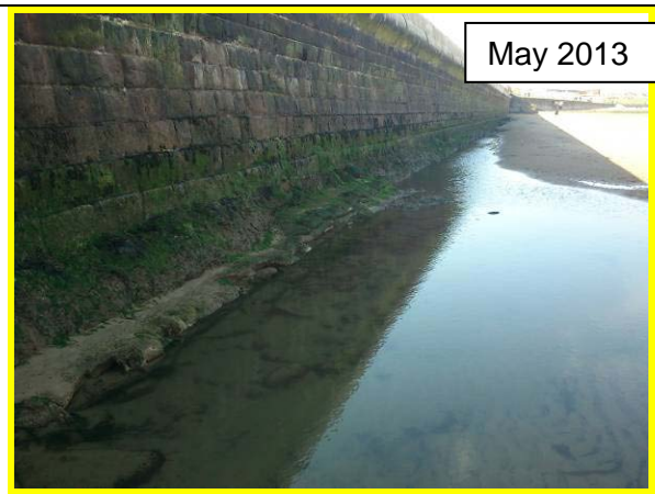
Low beach level in May 2013 exposing seawall toe which is undercut in places and previous concrete bagwork repairs (Asset ref. No. 121AB901B0603C03)
