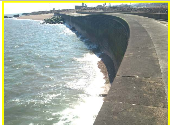
View of front face of wall 16.05.2013 (Asset ref. No. 121AB901B0801C03)
