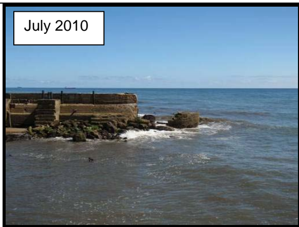
North East Pier failed roundhead July 2010 (Asset ref. No. 121AB901B0801C04)
