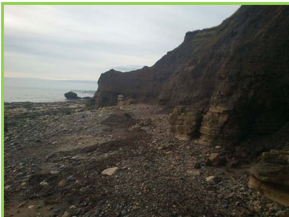
Multiple local mud slides in upper till slopes and arch formation south of Ryhope Nook. (Asset ref. No. 121AB901B0804C03)
