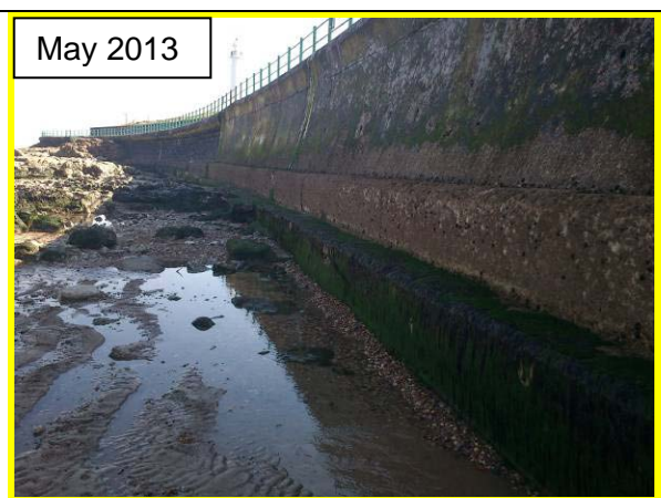
Low beach levels exposing lower section of wall in May 2013 (Asset ref. No. 121AB901B0604C01)
