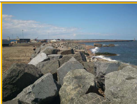
Stacked bund of rock armour at crest. (Asset ref. No. 121AB901B0801C05)
