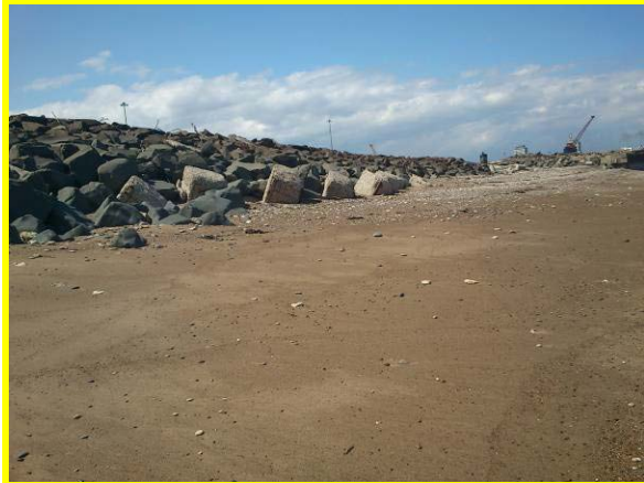
Northern section of rock armour (Asset ref. No. 121AB901B0801C02)
