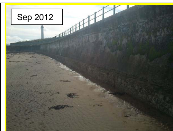
Seawall adjacent to Seaburn Park, showing chloride staining on surface of concrete encasement (Asset ref. No. 121AB901B0604C01)
