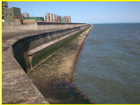
Spur barrier wall (Asset ref. No. 121AB901B0802C04)
