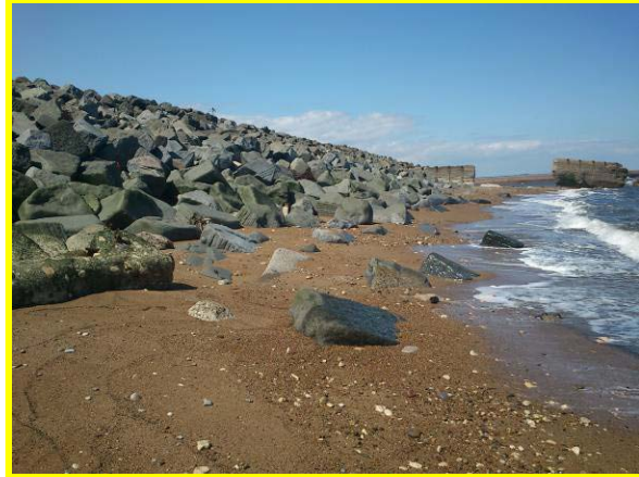
Southern section of rock armour (Asset ref. No. 121AB901B0801C06)
