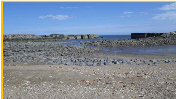
Looking seawards from South Outlet (Asset ref. No. 121AB901B0801C07)
