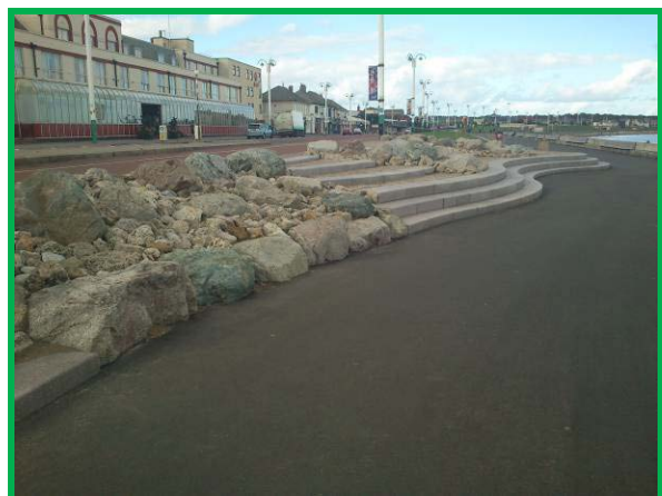
New promenade surfacing and rear revetment structures (Asset ref. No. 121AB901B0603C03)
