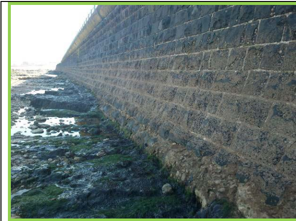
Masonry wall at Parsons Rocks (Asset ref. No. 121AB901B0604C02)
