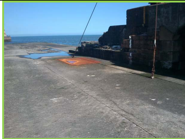
Internal access chamber cover has been repaired since 2010. (Asset ref. No. 121AB901B0703C01)
